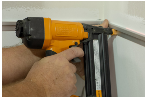
16-18 gauge 1" nails used to hold trim
