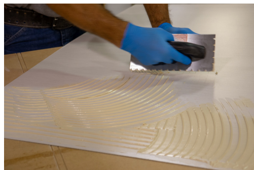
Apply adhesive. 100% adhesive coverage required.
