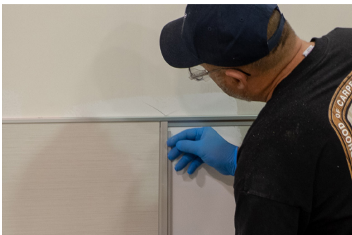
Install next trim
