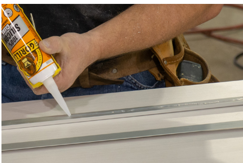
Use 100% clear silicone to adhere trim
