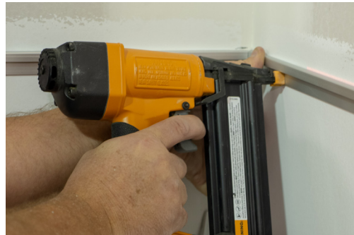
16-18 gauge 1" nails used to hold trim
