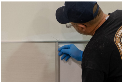
Install next trim
