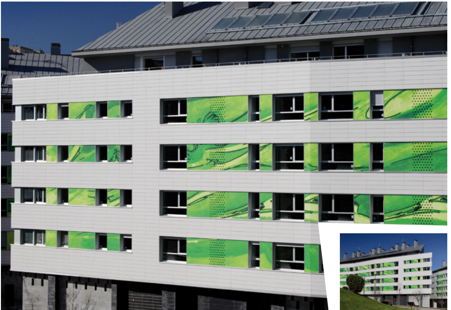
Miribilla residential buildings. IMB Arquitectura.
